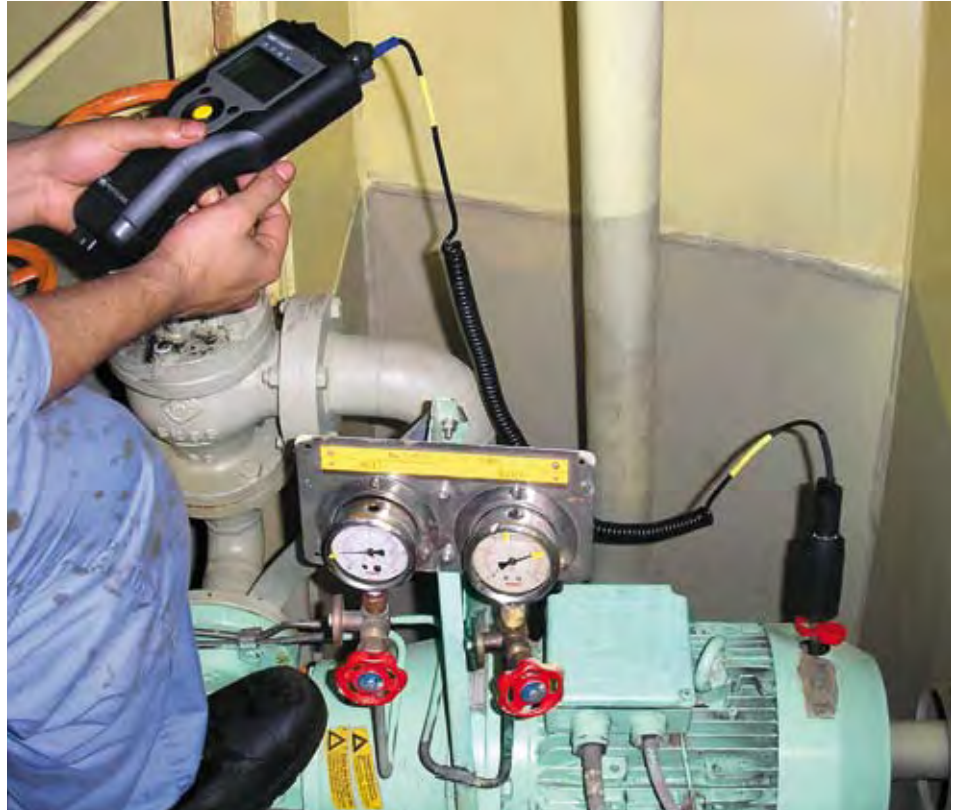
Routine monitoring of equipment can reveal important machinery health data
